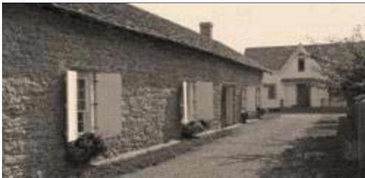
The Sifton-Cooke Heritage Centre on Orr Street
